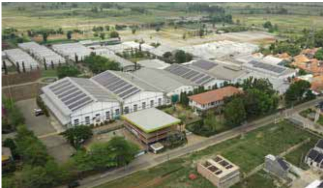
Indonesia: solar rooftop installation. © Xurya Daya Indonesia.
