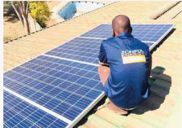
Photo: Zonful; solar panel installation.
