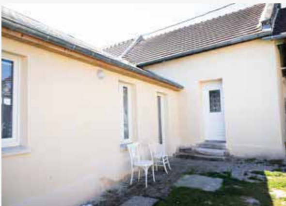
Photo: Réseau Eco Habitat; house before and after renovation.
