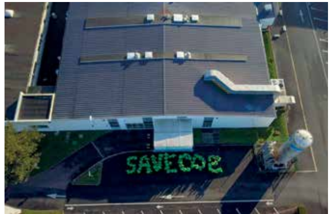
Schneider Electric’s Bourguebus site, France
